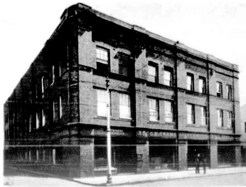
Head Office and Showrooms, 53 and 35 Pitt and Underwood streets, Sydney.
