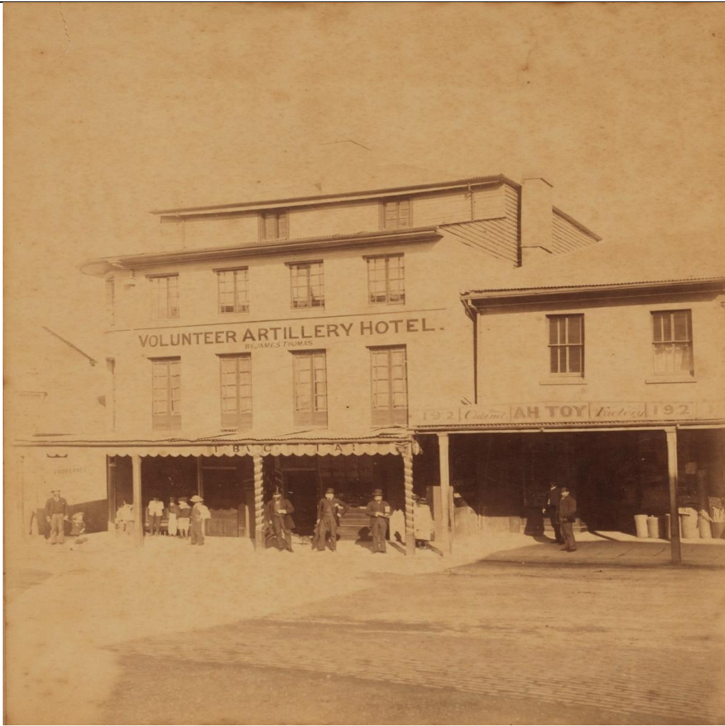
Ah Toy's Cabinet Factory, 192 Lower George Street. Date: c.1885 Source: State Library of NSW, https://collection.sl.nsw.gov.au/record/1JkmAW5Y/8re5BkaGP2ALz
